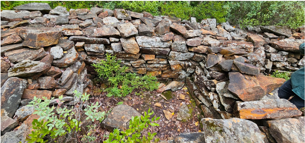
A section of the Bayers Lake Mystery Walls, built from stacked quartzite, slate, and granite slabs.
